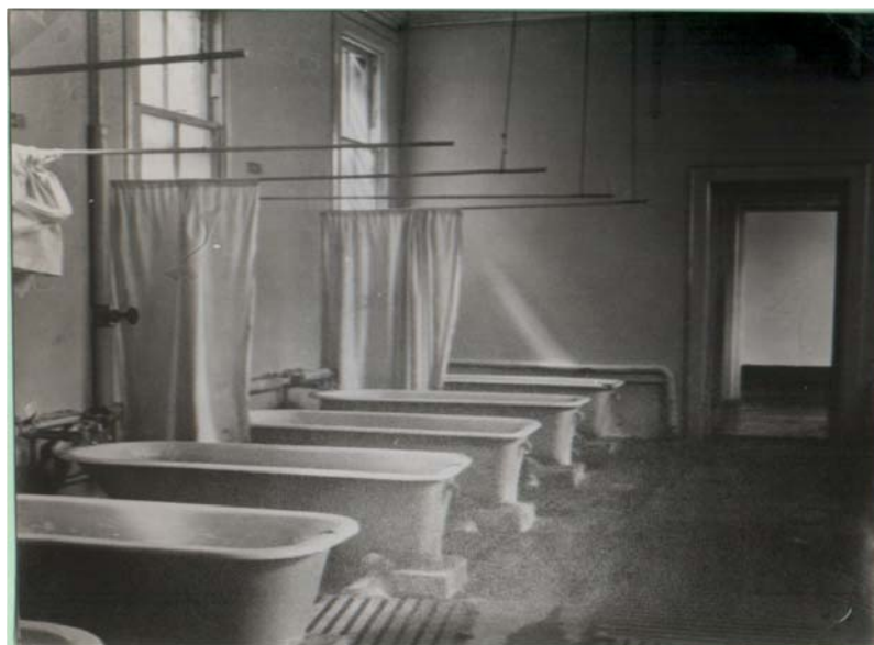
Figure 14. Bathrooms, F6, Oakley Hospital before renovation, 1960. Source: Personal collection.
