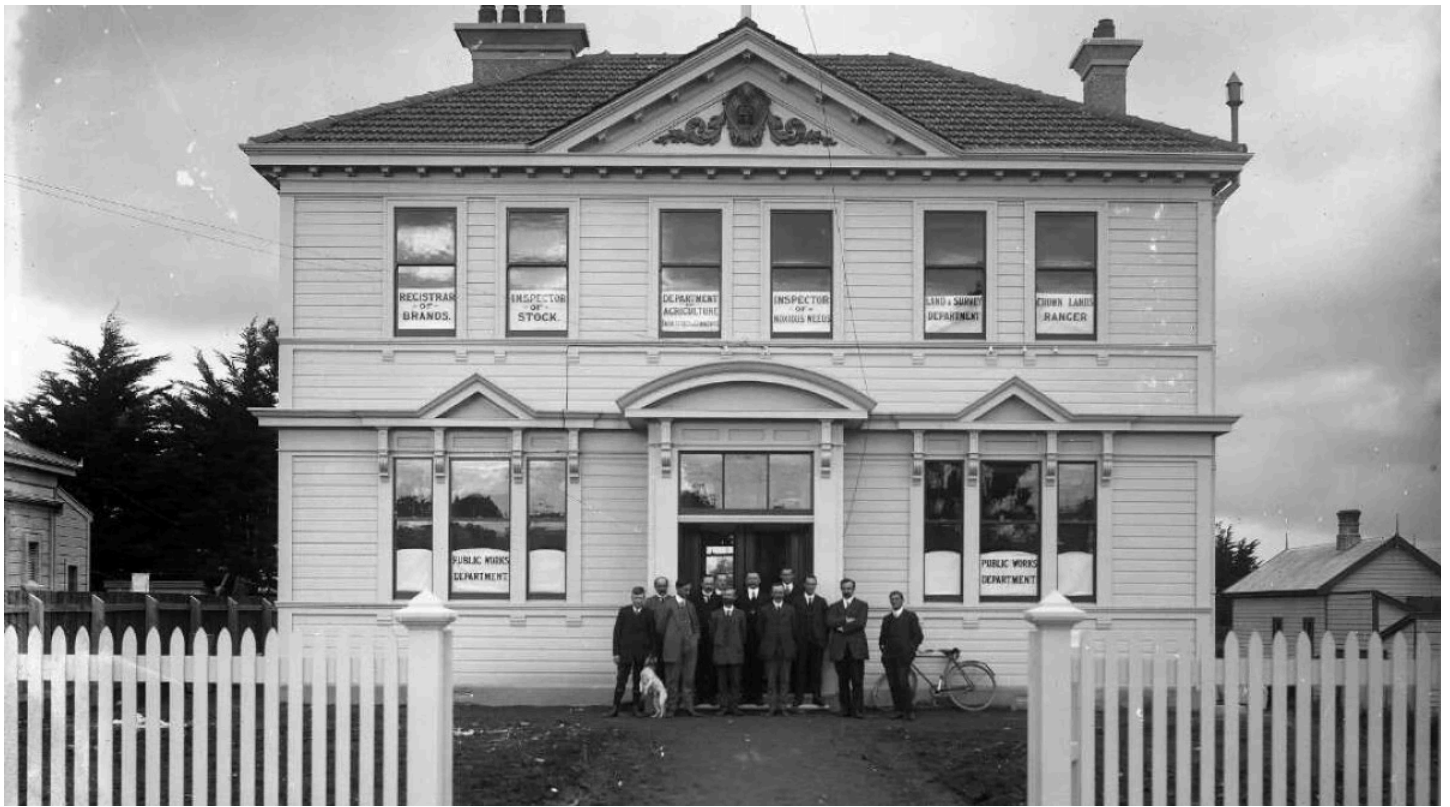
Government department building in Stratford with employees of the Public Works Department standing outside in 1913. McAllister, James, 1869-1952 :Negatives of Stratford and Taranaki district. Ref: 1/1-009395-G. Credit: Alexander Turnbull Library, Wellington, New Zealand. https://natlib.govt.nz/records/22904136
