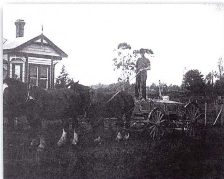
FIG 3.2 Mr G Reynolds outside Mr W Melville's house on the corner of Mangapiko Street, Te Awamutu with his team of horses and load of sand for Tokanui buildings. In the years 1910 – 1912 Mr George Reynolds with his team of horses carted the metal and timber and sand to Tokanui to build the Superintendent's house and the hospital. The first of the hospital buildings was finished and the patients moved to their new home in July 1912.
