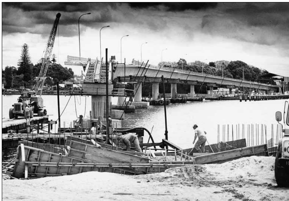
Figure 6.1: Tauranga Harbour Bridge under construction, 1987
